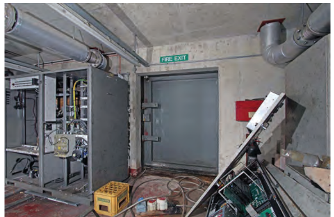
The machinery entrance blast door
